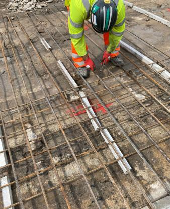
The team also discovered that the centreline crown and the camber that creates a fall to both kerb lines was not formed by asphalt, as first thought, but by the bridge deck itself, requiring precision concrete to be installed at various different levels.
