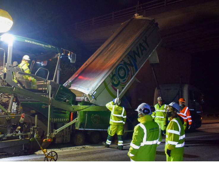
The innovations used in developing the new materials have driven substantial carbon savings. The high RAP content resulted in a 23% reduction in carbon compared with traditional materials, while manufacturing the asphalt as a warm mix saved a further 14% as it only had to be heated to 150°C. Standard hot mix asphalts are heated to 180°C.
